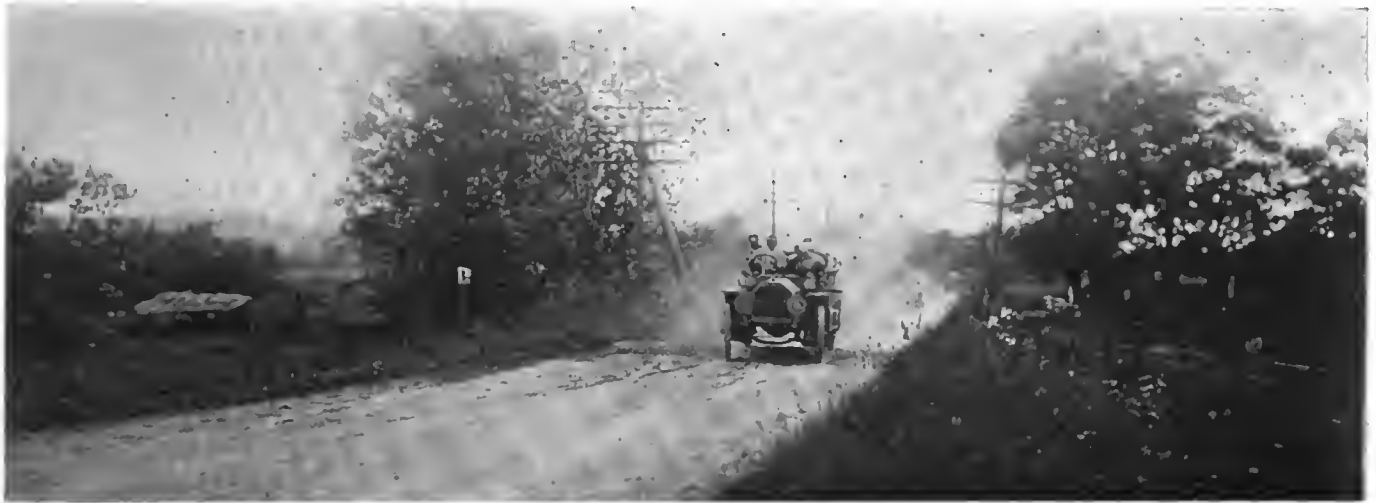
BURMAN (PEERLESS) TACKLING 1863 WATER BREAKS OR "THANK-YOU-MA'AMS" THAT CORRUGATE PENNSYLVANIA ROADS.
